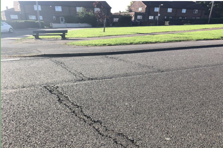
Joint Failure
