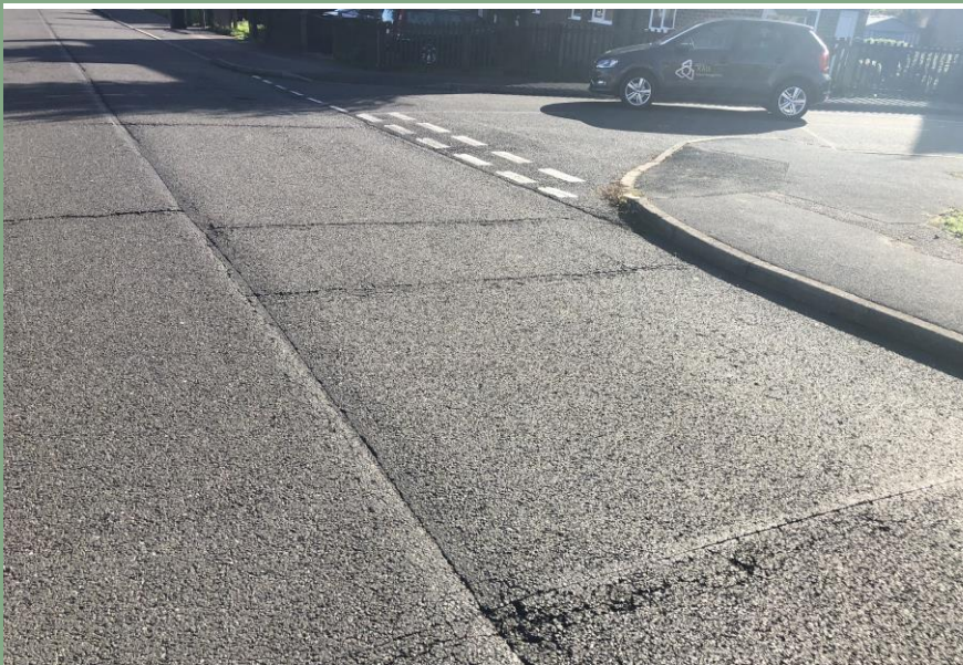
Joint Failure
